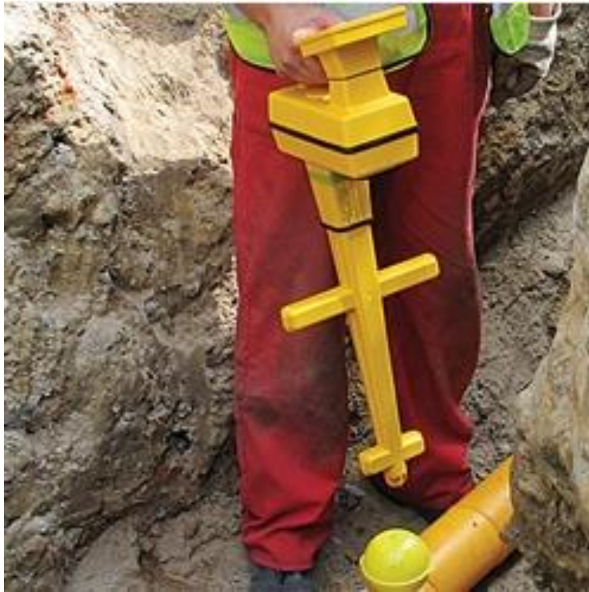
Figure 8-52 Installation of marker ball
