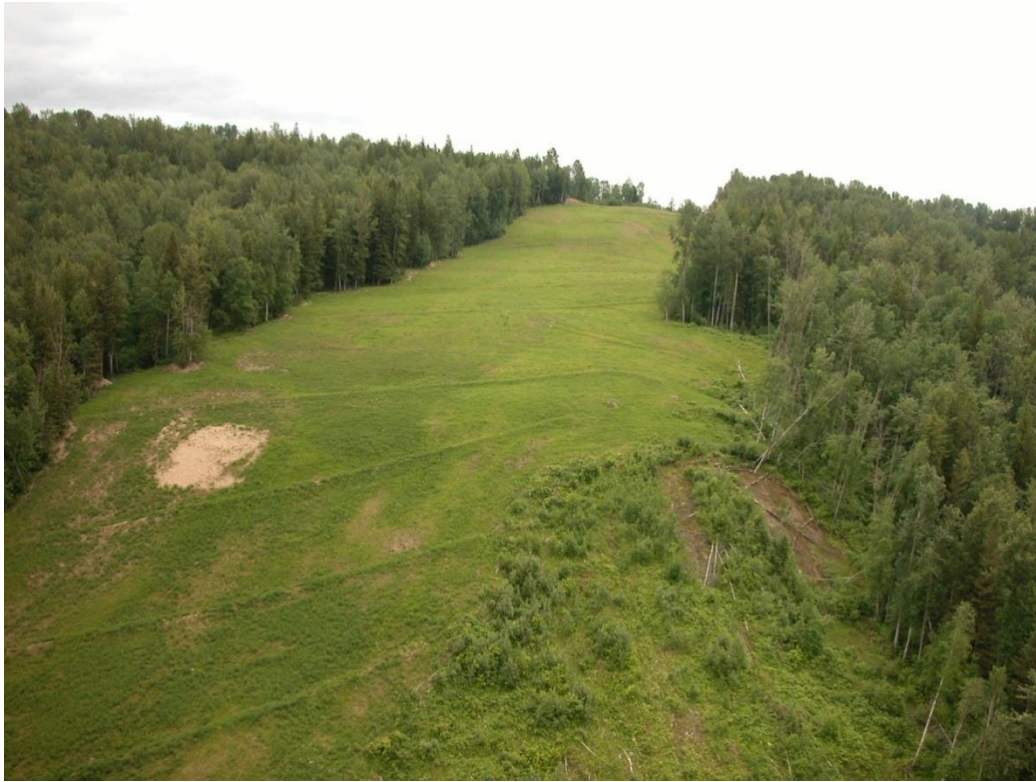
Figure 8-13 Surficial water diversion berms (slope breakers) on ROW (Location: Central British Columbia, Year: 2011)
