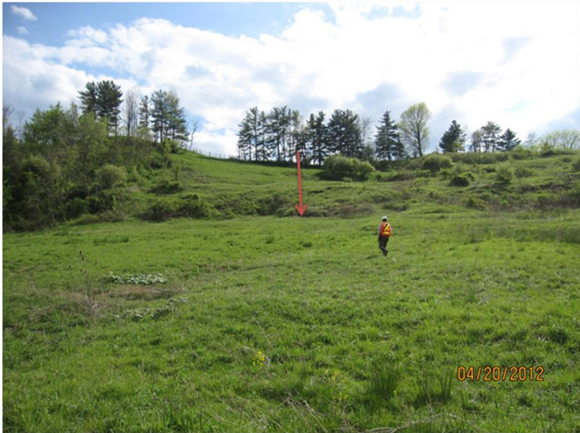
Figure 2-57 “High” threat level landslide G-417 with pronounced toe (at arrow), that disturbs the ROW and has geomorphic evidence of movement less than 10 years old.
