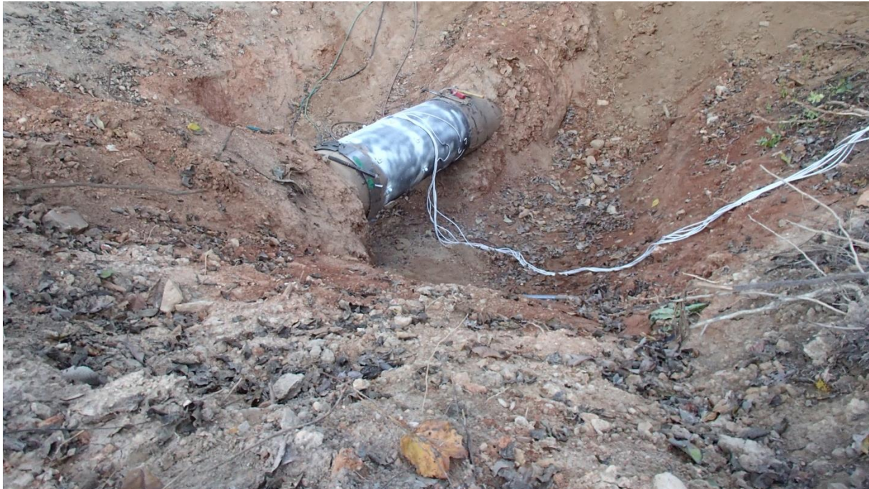
Figure 8-79 A site with resistance type strain gauges installed
