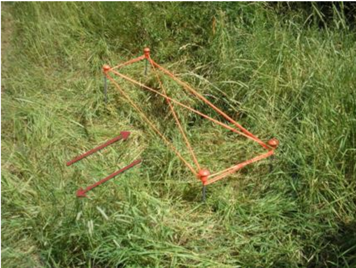
Figure 8-29 View of a rebar quadrilateral array across a landslide lateral scarp (lateral scarp location and relative movement shown by arrows) (Photo by: D. West, Year: 2010)
