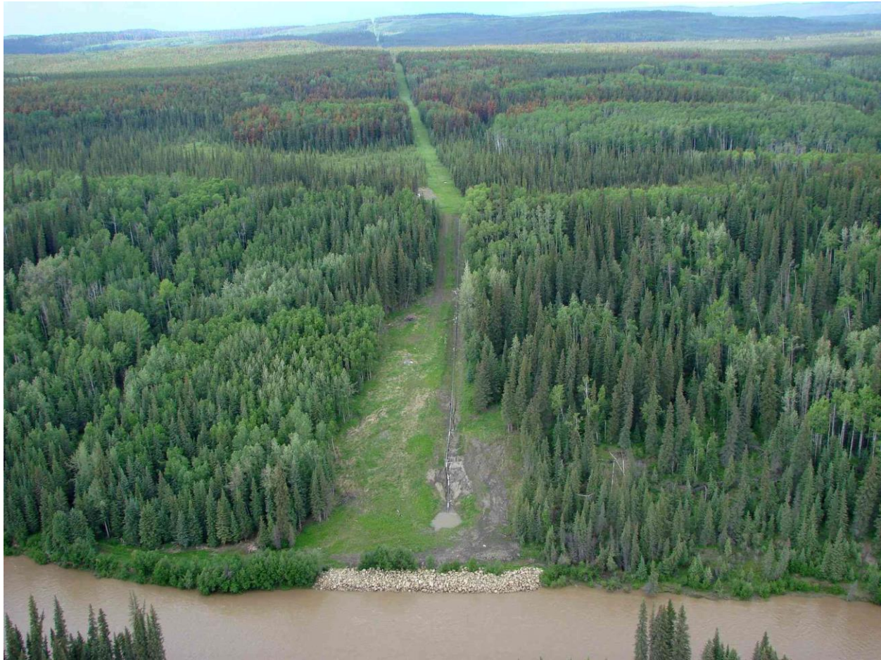
Figure 8-4 Surface pipeline segment running parallel to the direction of movement (Photo by: L. Allen, Location: Northwestern British Columbia, Year: 2011)
