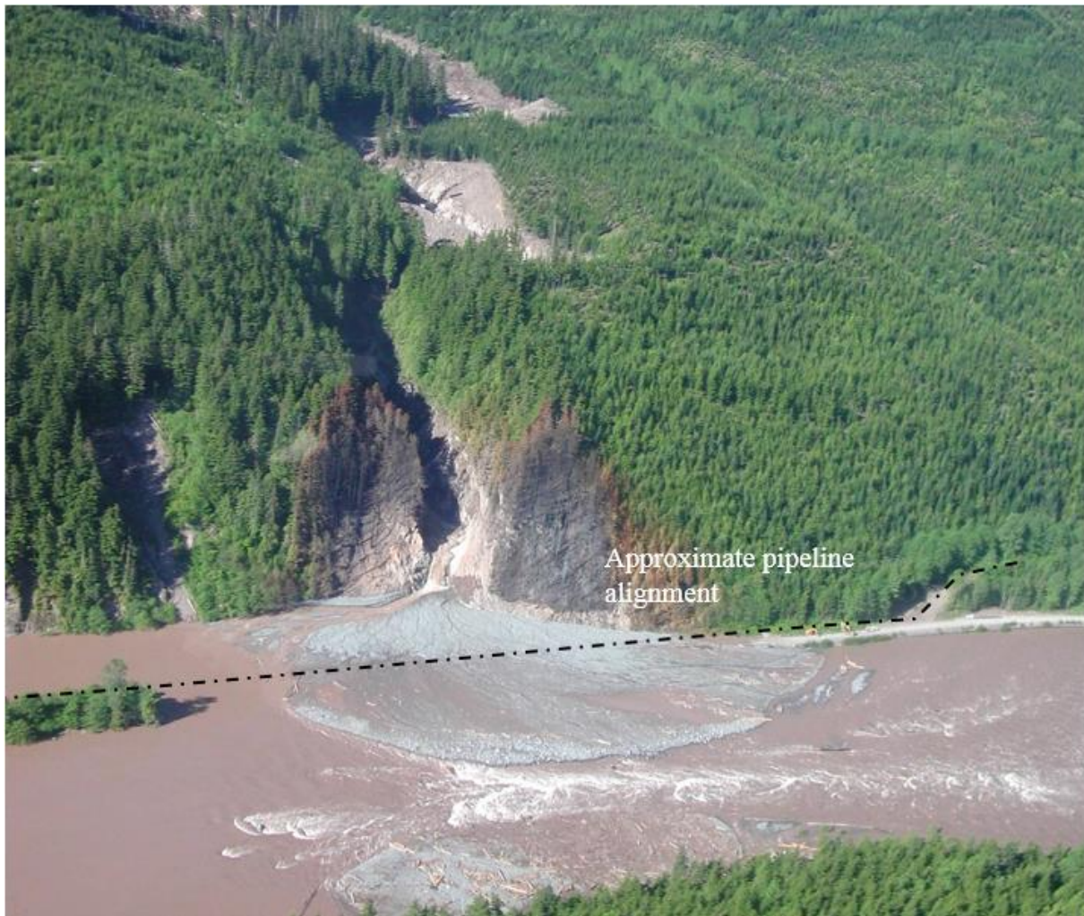
Figure 2-34 Pipeline rupture on a 16-inch natural gas mainline, which is routed along the toe of a mountain slope at the Zymoetz River, as a result of a debris flow. Rupture occurred during the initial scouring of the existing alluvial fan, during the initial stages of the event and prior to deposition of debris. Note the extent of the burned area as a result of the rupture and ignition [68].
