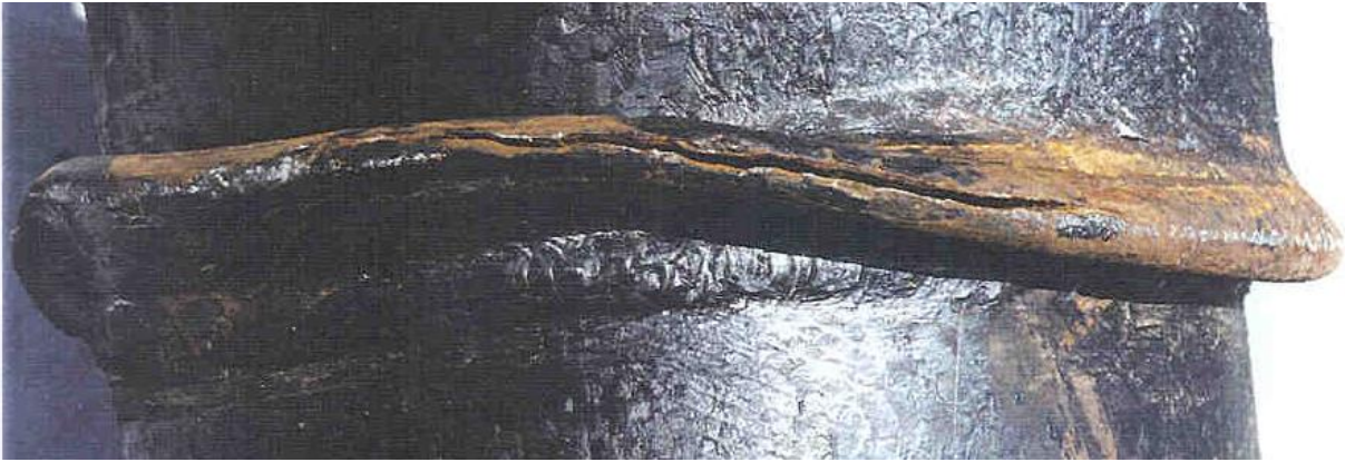
Figure 1-9 Wrinkle formation near a girth weld and the resulting cracking of pipe wall at the apex of the wrinkle
