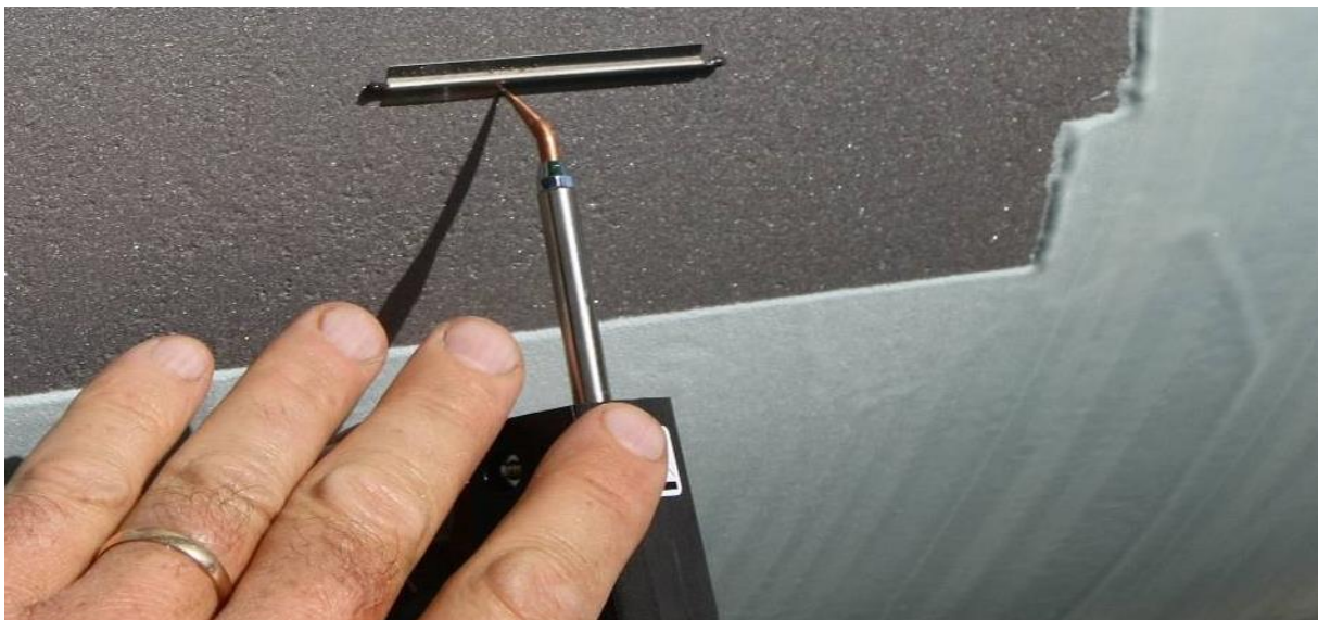
Figure 8-81 VW Strain gauge in the process of being spot welded at 3 o'clock position on a pipeline (Photo by: D. Dewar, Year: 2004)
