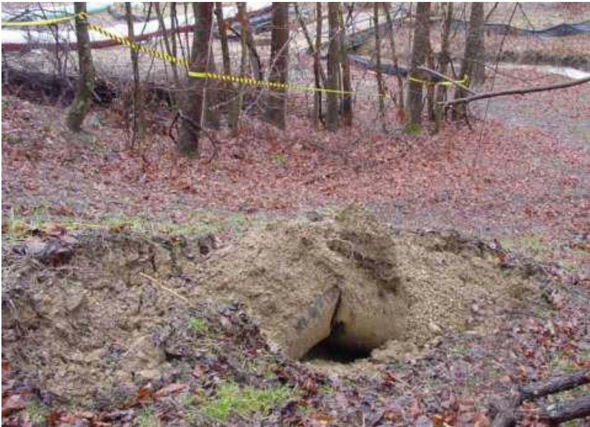
Figure 1-7 A severe buckle formed at zero internal pressure.
