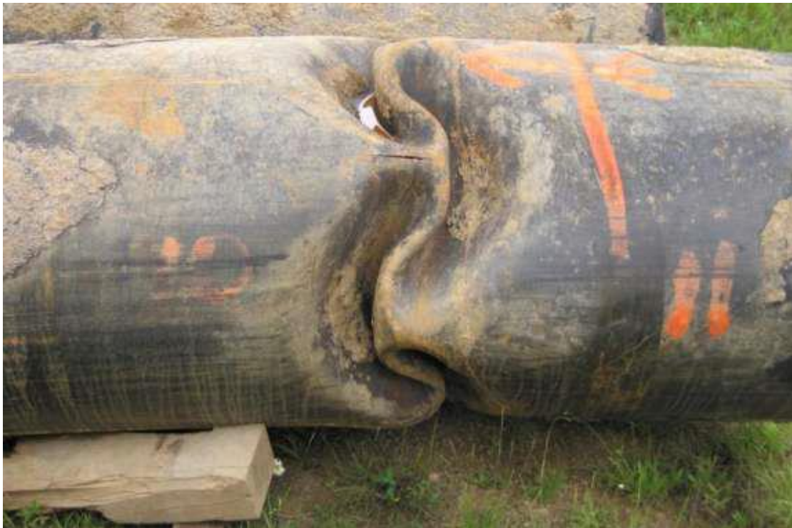
Figure 1-6 A severe wrinkle formed at zero internal pressure.
